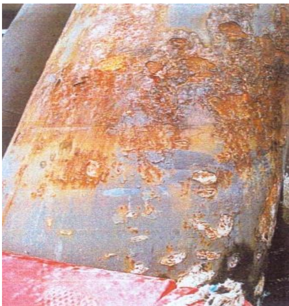
Fig. 62: Coating damage in tidal zone [27].
