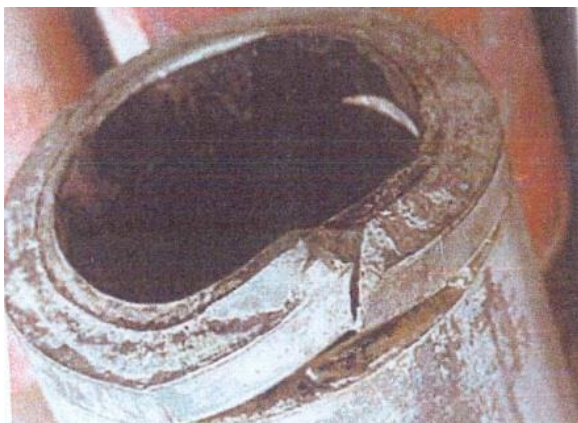
Fig. 69: Oil and gas pipeline under sour (under hydrogen sulphide and moisture) corrosion [28].
