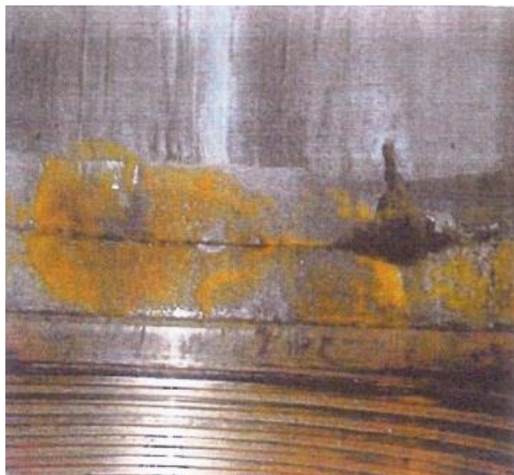
Fig. 64: Oil and gas pipeline under crevice corrosion [28].
